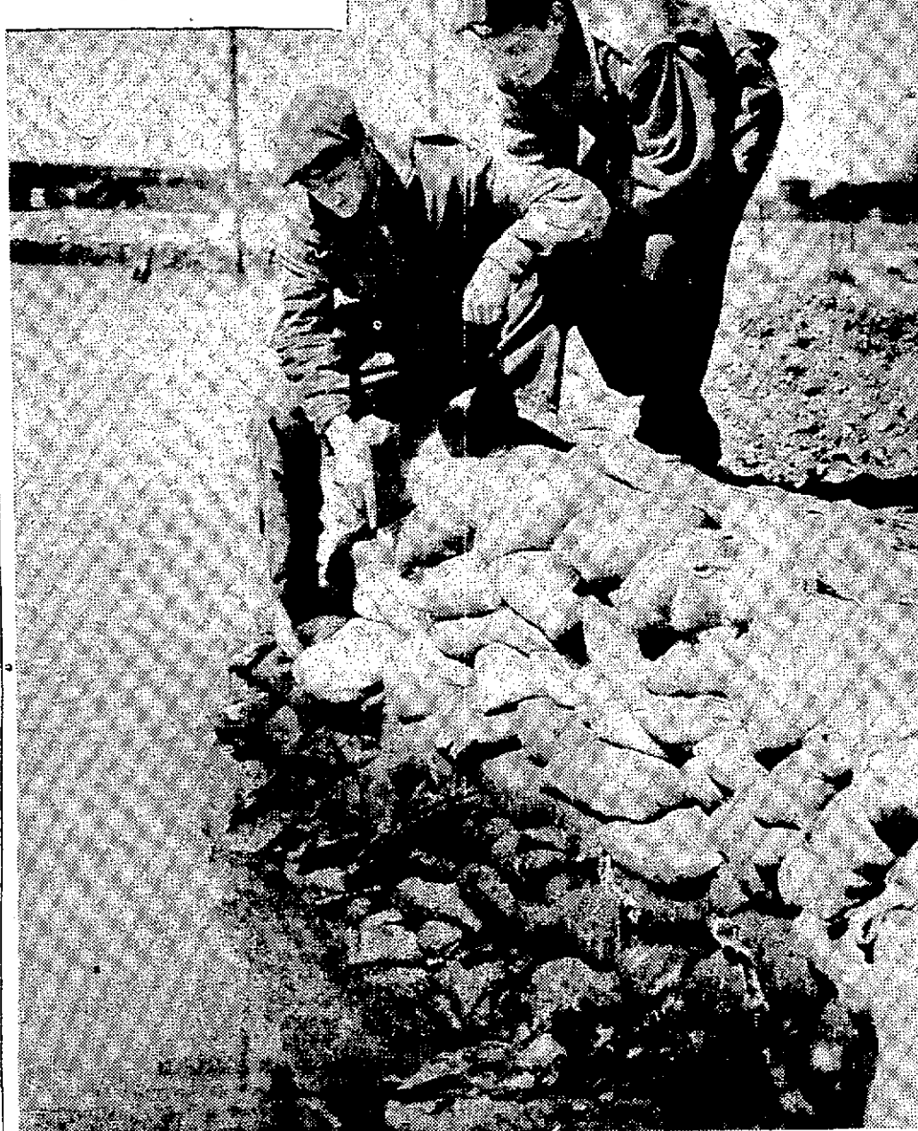
High-water mark on soggy sandbags making up part of the Lyndale dike is now two feet above the present river level. Here, from left to right, Pte. Archie Reid and Pte. P. J. Trembley, both with the P.P.C.L.I. from Calgary, Alta., are ready to check the peak height against the present level.
