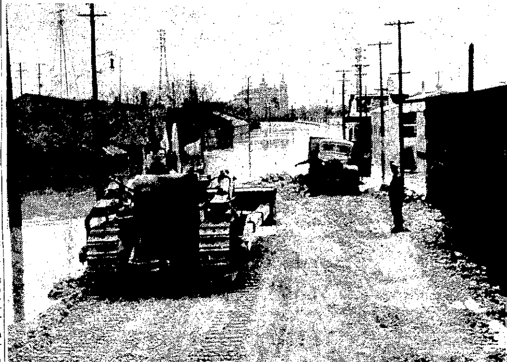
Workmen are pouring thousands of tons of gravel into an improvised ramp to Provencher bridge in an effort to build up and re-open it to traffic. A bulldozer here packs down gravel on Water avenue. The water gap yet to be filled is 250 yards long.
