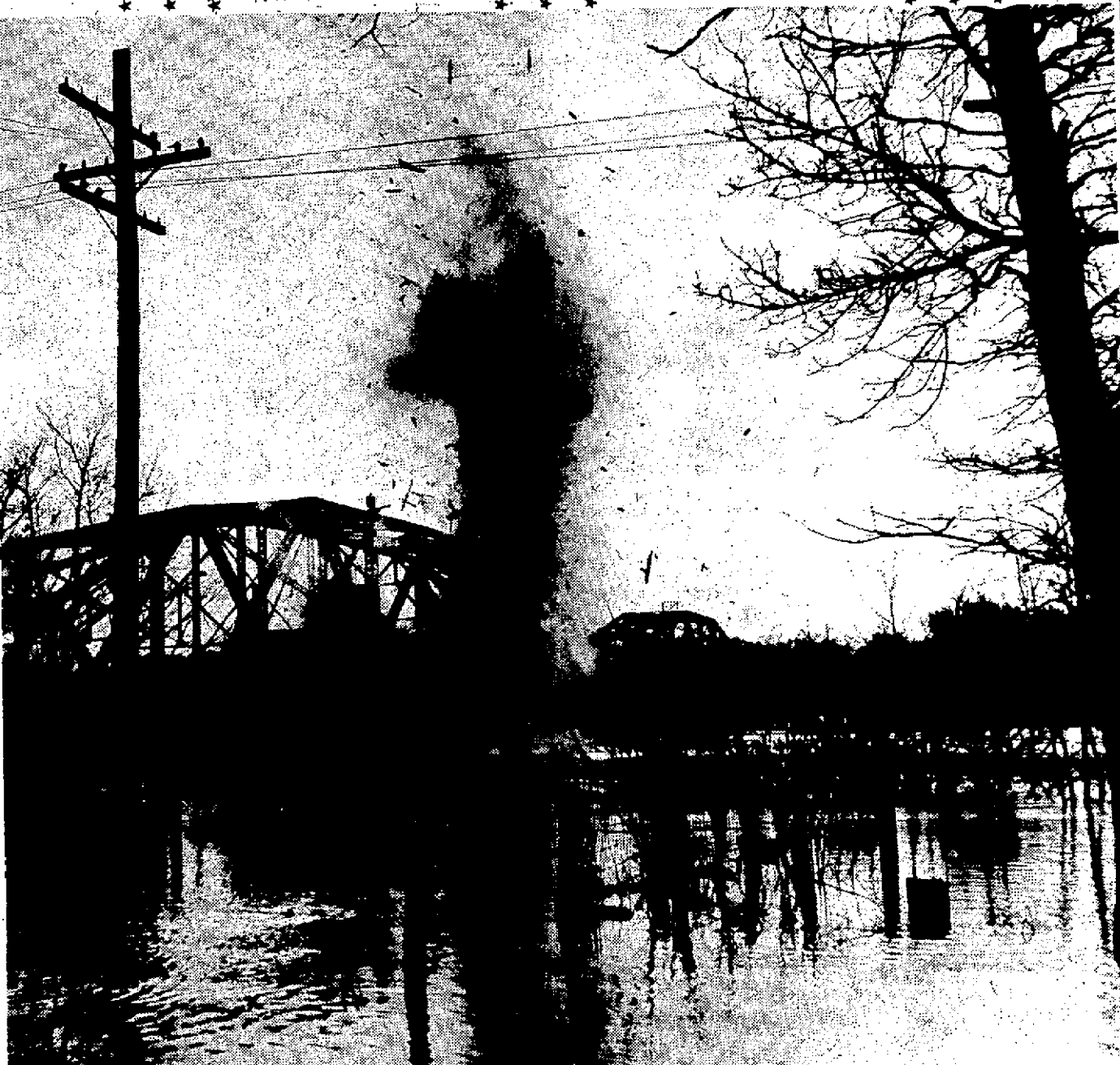
Blasting operations were underway at Elm Park bridge Monday. At first glance, it would appear that the twin-spaced steel structure itself is on its way to Davey Jones' locker at the bottom of the murky Red river. However, the object of the blast was to unloose the roof of a summer cottage which had lodged against the bridge. Four two-pound charges of "gun-cap" were placed in the corners of the cabin, and other charges were laid among surrounding debris.
